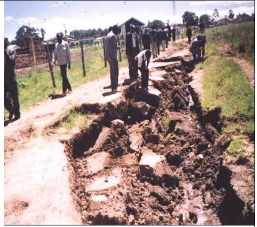
Figure 5. 7. Gully formation and soil erosion along access road to Bomet Town, upstream of 1LA03.
