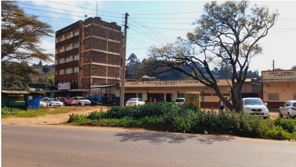
Figure 4.29: Maziwa House, Animal Feeds and Pyrethrum Board buildings
