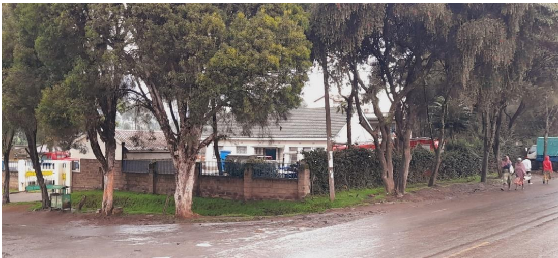
Figure 4.40: Molo Sub-County Offices with Live Fence Hindering Visual Access
