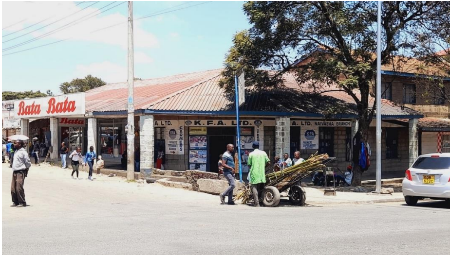
Figure 4.36: Good Visual Access of the KFA Building in Naivasha
