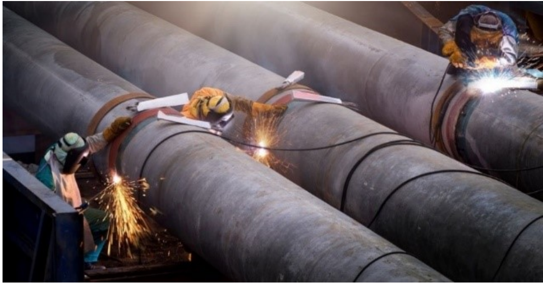
Figure 1.1: Pipeline Welding (Phillips et al., 2022).
