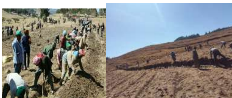
Figure 3: Stone-Faced Soil Bund Constructed by the Community Mobilization
