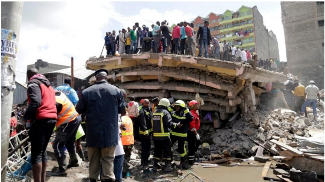
Figure 1.1: Rescue Operation after a Building Collapse in Nairobi on 6 th December 2019
