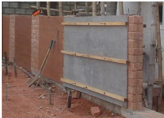
Figure 2.5: CSRE Boundary Wall in a Residential Building
