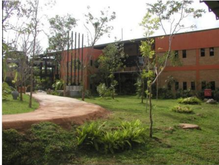
Figure 2.6: Driveway Completed with CSRE
