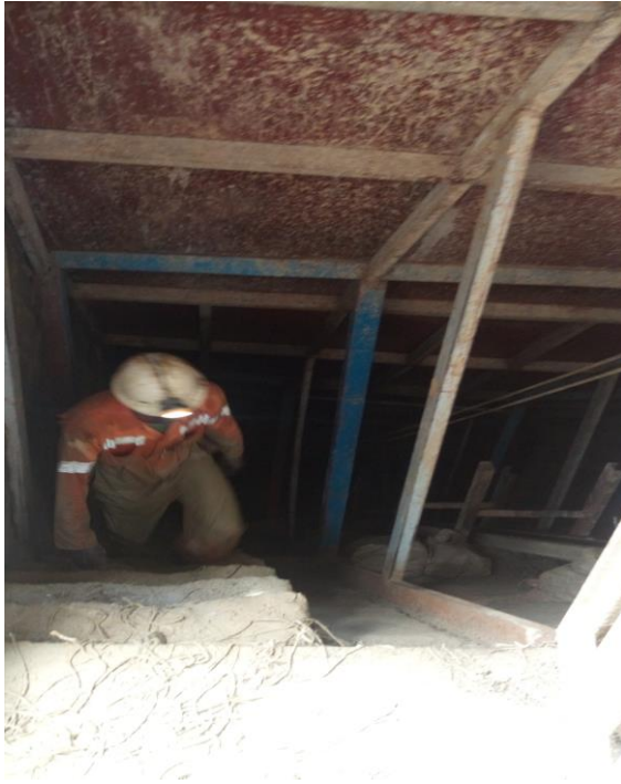
Plate 4.2: Working Underground with Limited Lighting Using Torches and Ventilation Systems
