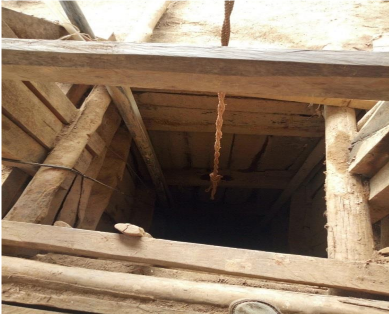
Plate 4.3: Construction of Underground Mine
