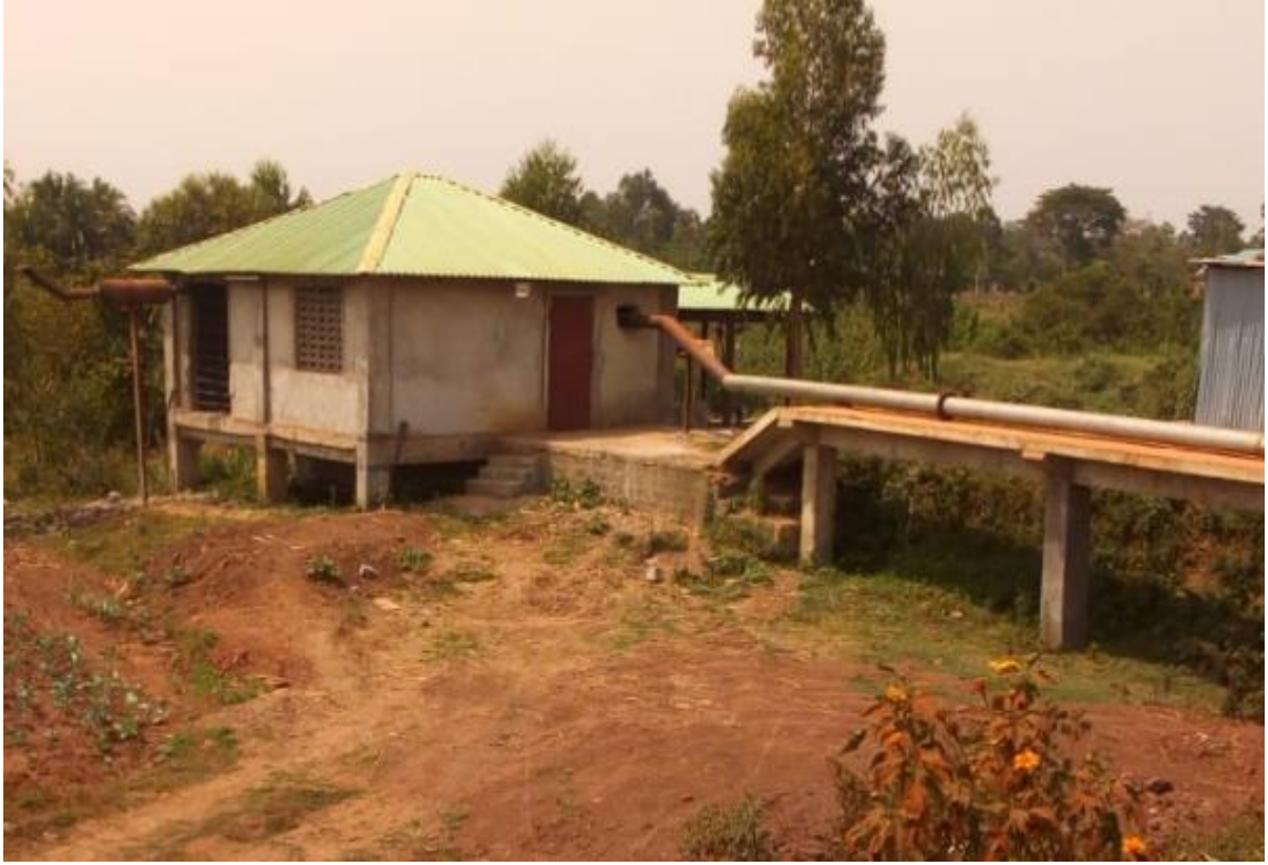
Plate 3.2: Water abstraction station used by Busia sugar industry at the banks of River Sio (Source: author)
