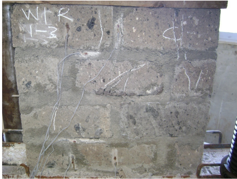
Plate 8.1: Cracking pattern for reinforced conventional block wall utilizing 1:3 jointing mortar
