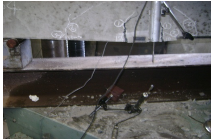
(b) Final cracks pattern at ultimate load
