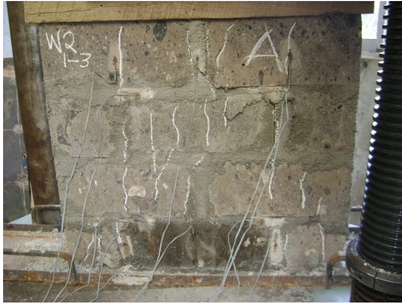
Plate 8.2: Cracking pattern for plain conventional block wall utilizing 1:3 jointing mortar
