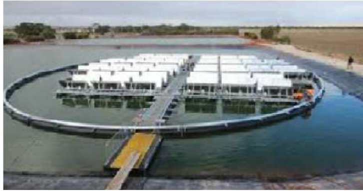
Figure 2.7: 4MW Tracking type floating system Jamestown Australia (Divya Mittal et al., 2017)
