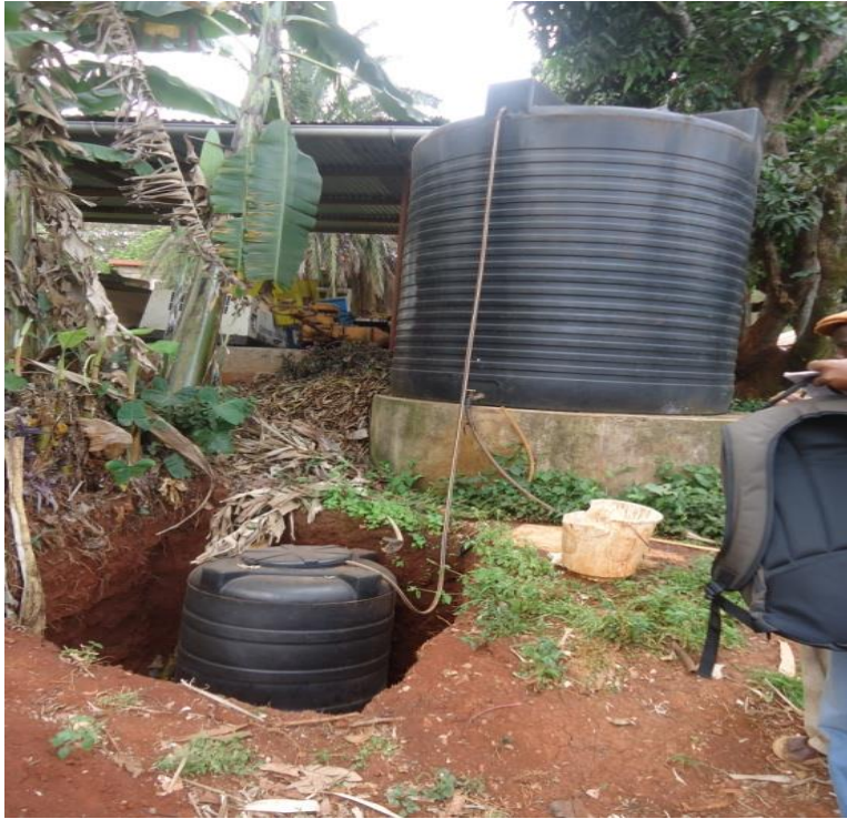
Plate 4. 7: Roof-water harvesting technology at Umoja Estate in Embakasi Sub County, Nairobi County, Kenya. (Source: author, 2014)
