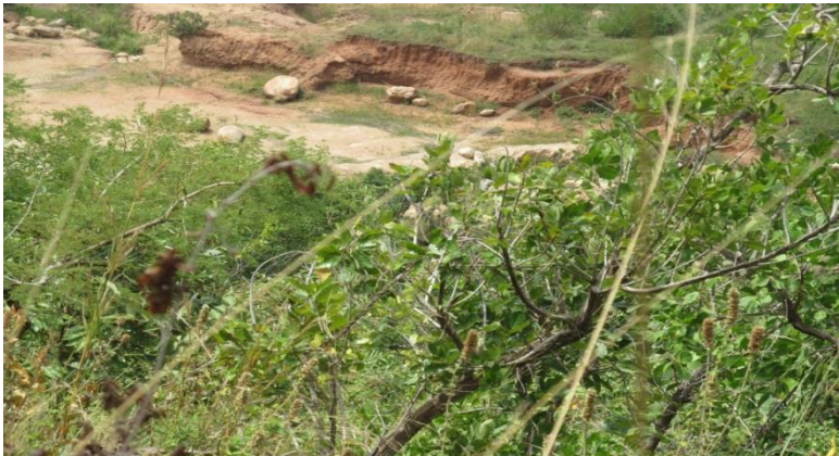
Murram excavation; Photo by Daniel Mokaya
