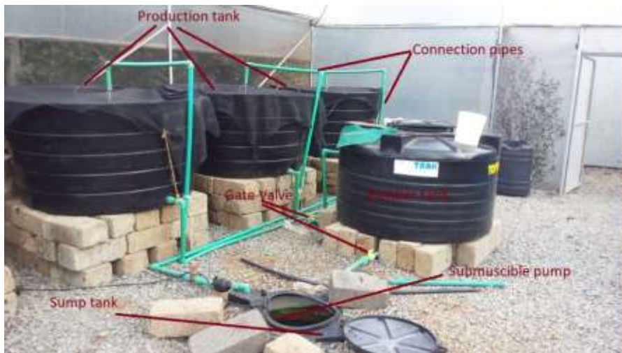
Figure 3.2: The RAS Production Tanks, Biofilter Tank and Sump Tank among other Components
