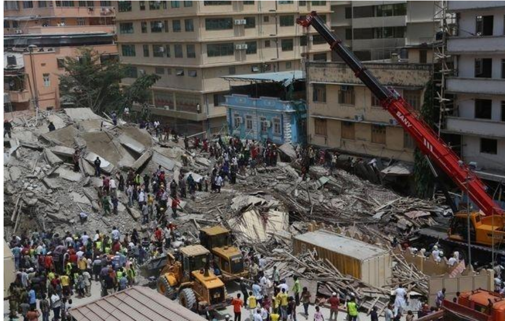
Figure 2.5: A 16 Storeyed building collapsed in Dar es Salaam in 2013
