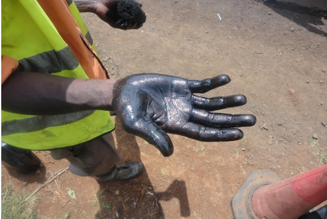
Plate 4.6: Exposed hands of an unskilled labourer on Marua – Karishen road. No PPE (gloves) provided
