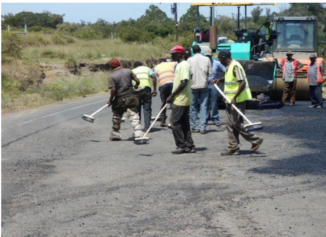
Plate 4.1: Workers not in the required work-gear (PPE) on Nyeri – Wiyumiririe road
