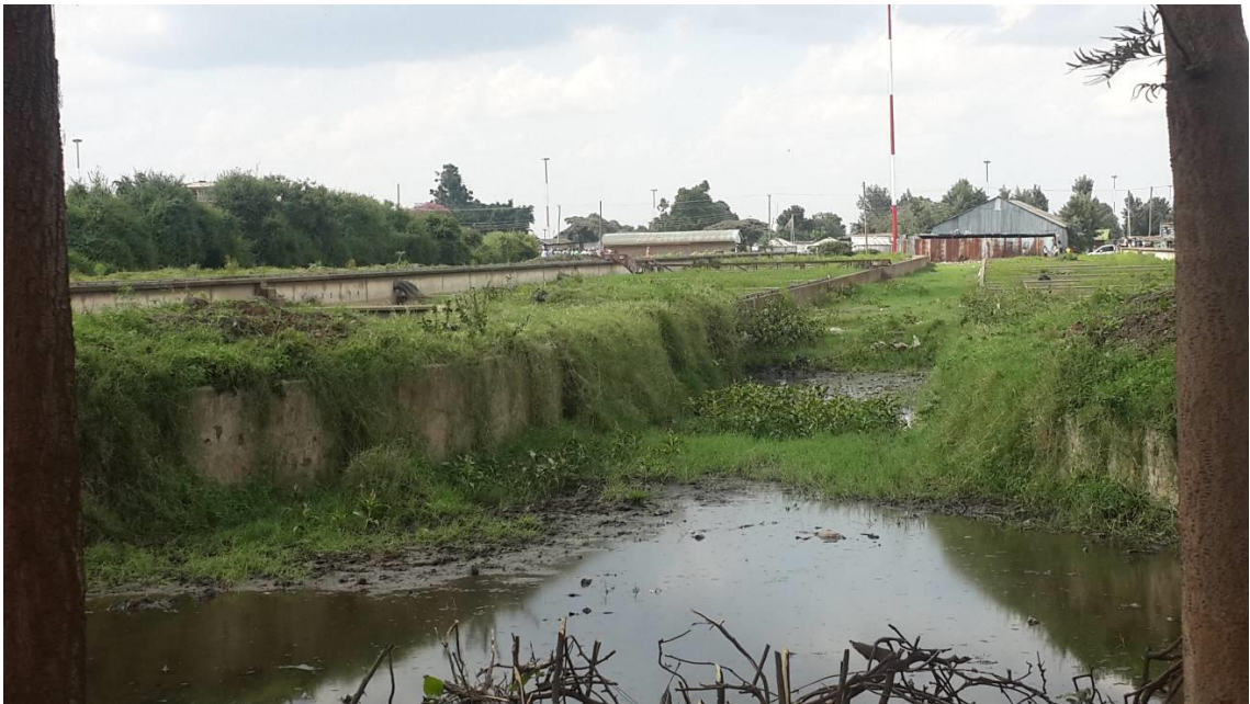
Appendix II: Kariobangi sludge drying bed
