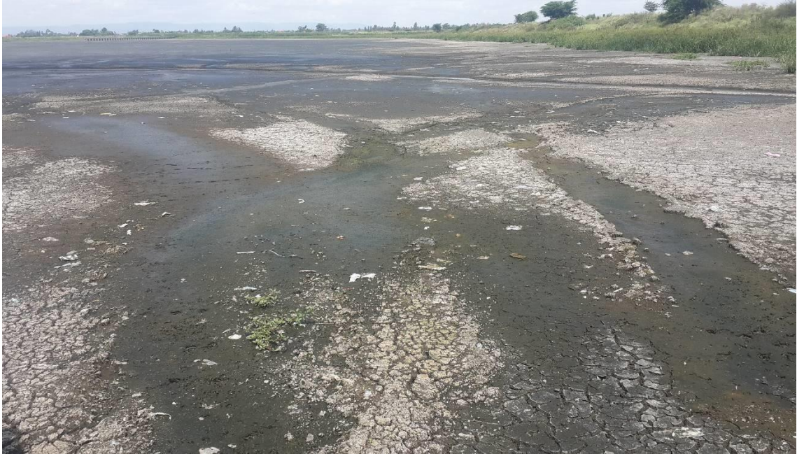
Appendix I: Dandora sludge drying bed
