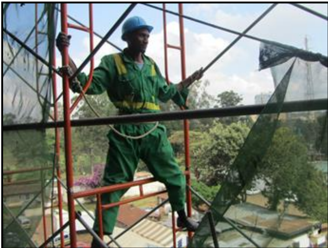
Figure 4.3: Use of safety rope while working at heights in Westlands
