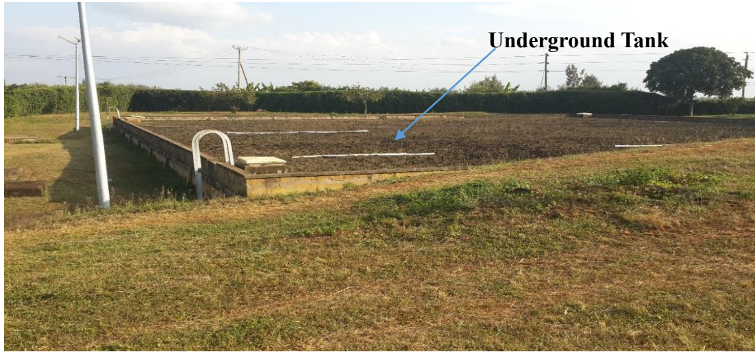
Plate 3.2: Treated water storage reservoir at Ng'ethu
