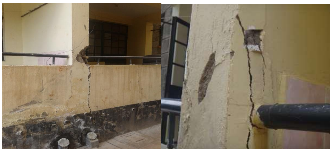
Figure 2.22: Cracks in exterior walls for a building built on black cotton at Mavoko (Machakos County)
