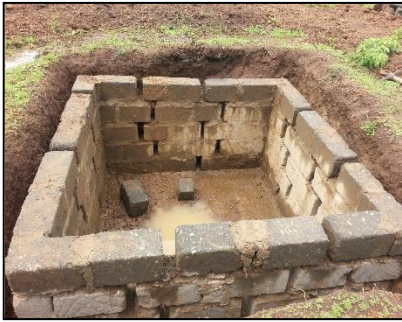
(a) Walling under construction
