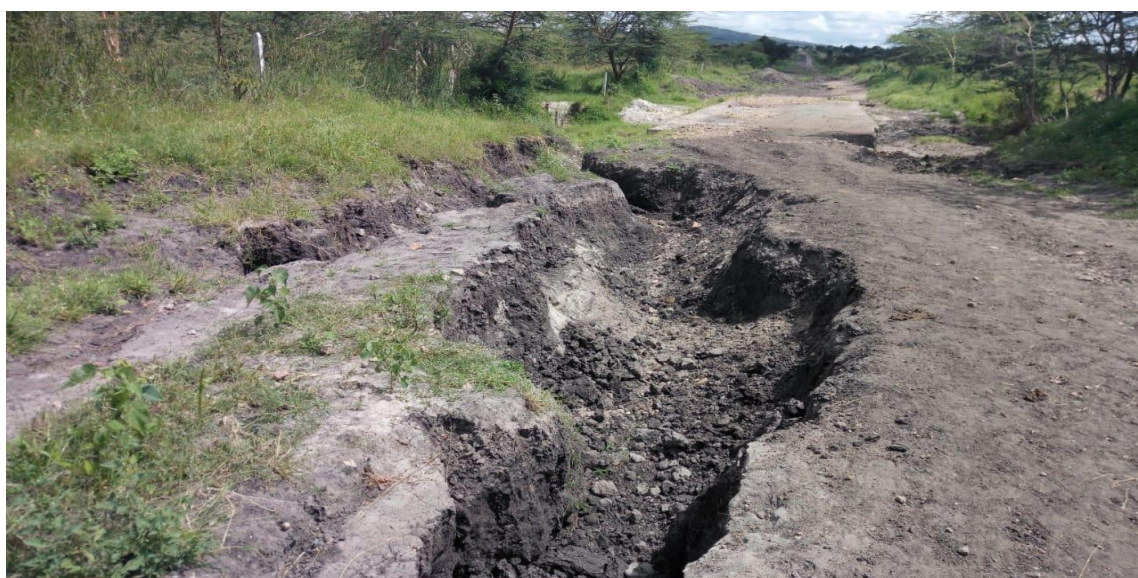
Figure 2.23: Extensive damage on a road on black cotton soil (Katumani-Vota-Konza Road, Machakos County)
