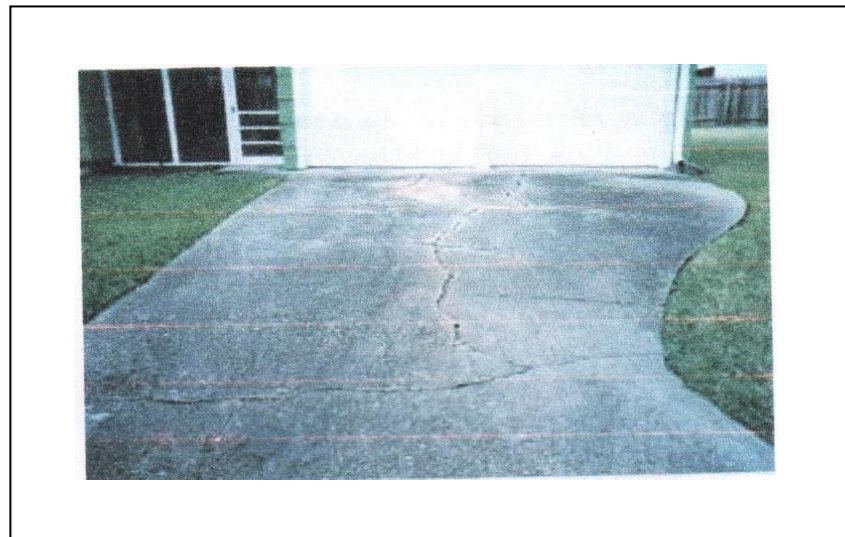
Figure 2.21: Residential driveway damaged by expansive soil
