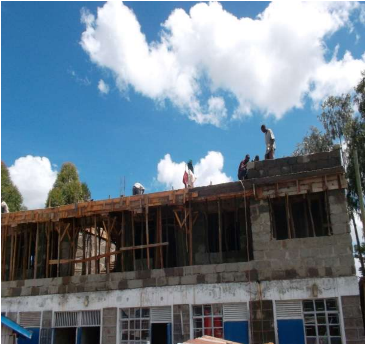
Plate 4: Storey building under construction in Shabaab, Nakuru
