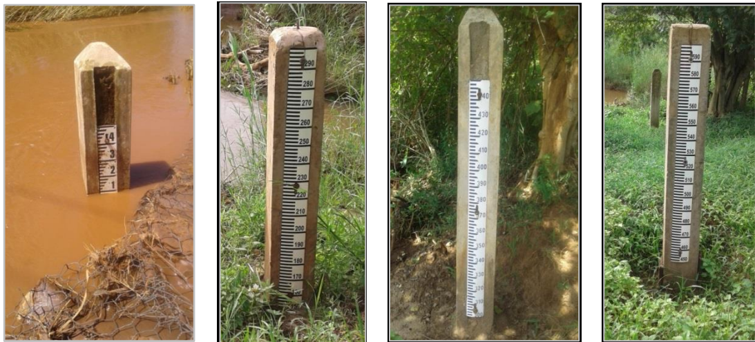
Plate 4.3: Four Flow Gauges of 3KG01 Gauging Station with their scales for measuring Water Level 0 to 1.5m, 1.5 to 3.0m, 3.0 to 4.5m, and 4.5 to 6.0m
