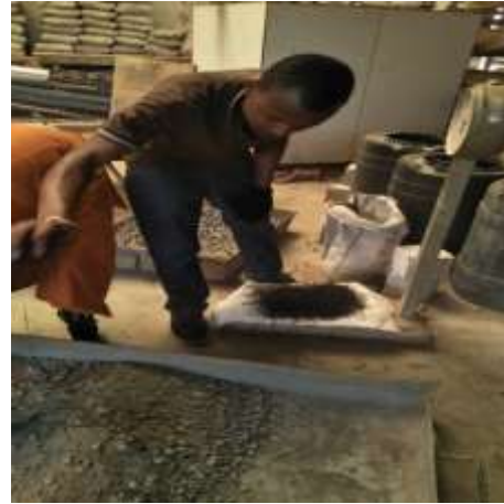
Fig.A-9-14. Adding the steel fibre in a mix
