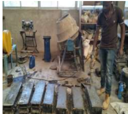
Fig.A-9-24. Casting of concrete beams
