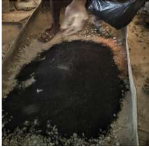
Fig.A-9-13. Adding Crumb rubber in a mix
