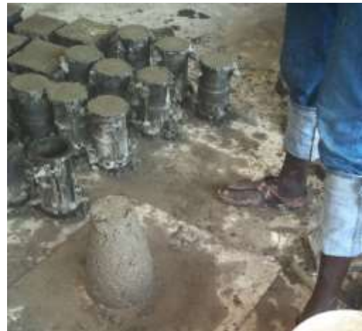
Fig.A-9-20. Casting of cubes and cylinders
