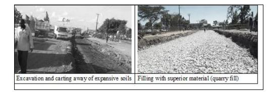
Figure 4.12: Cutting and filling activities during construction of Enterprise Road
