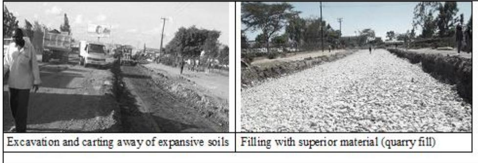
**Figure 4.12: Cutting and filling activities during construction of Enterprise Road**
