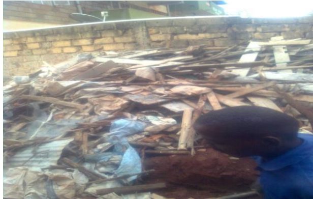
Plate 4.5. Off cut timber and roof coverings timber, concrete rubble dumped on site. Source: Field survey 2015
