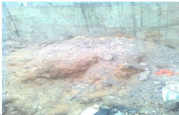
Plate 4.6. Sand mixed up with soil & damaged due to weather effects.
