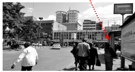
Plate 5.65: Old Nation House Building, 2015 Source: Author
