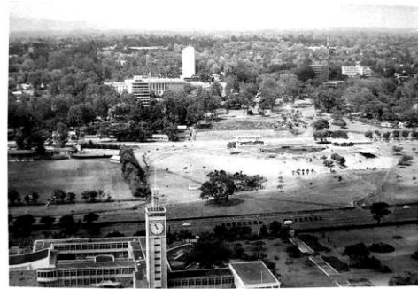
Plate 3.4: Containing Sprawl: Uhuru Highway and Uhuru Park, 1970s. Source: www.sikh-heritage.co.uk
