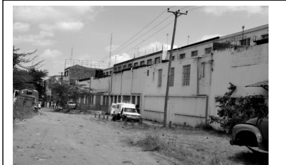
Plate 1.5: Low visual and functional interaction between buildings and park at John Michuki Park. Source: Author (2013)
