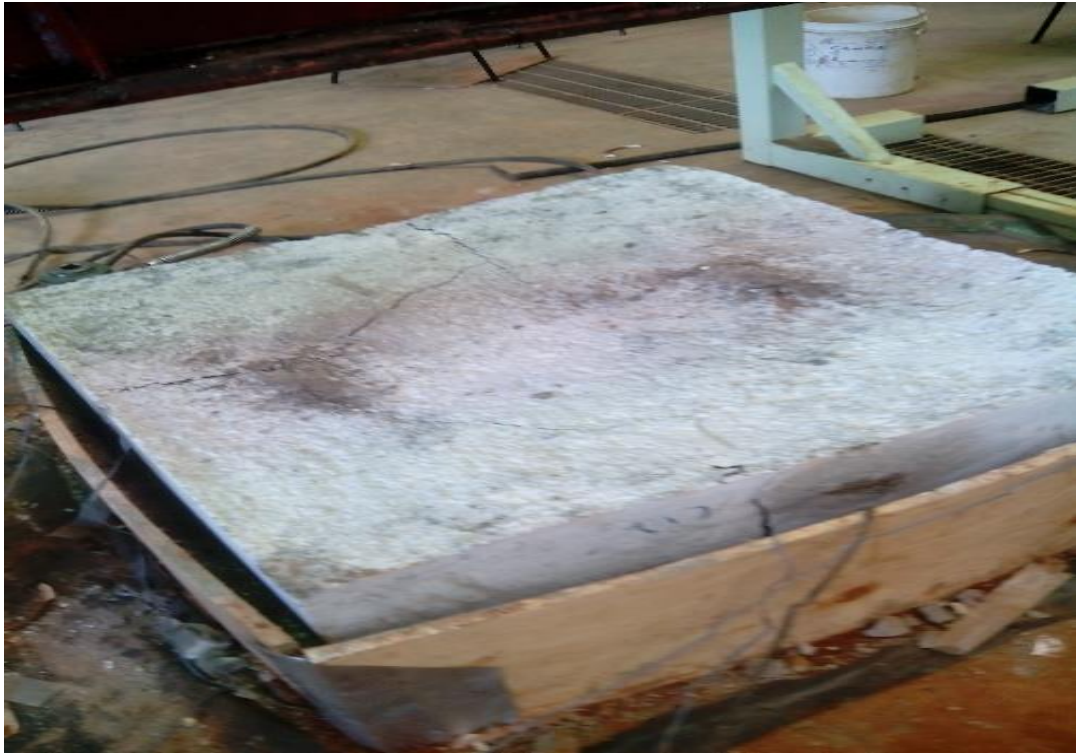
Plate 4.1: Cracks appearing all over the slab, an indication of uniform loading
