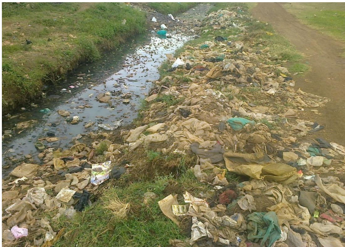
Plate 4.1: Open drain clogged with solid waste
