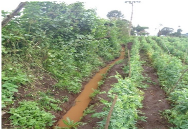
Plate 4.3: A retention ditch (capturing water from rural rough roads) (source: author, 2016)
