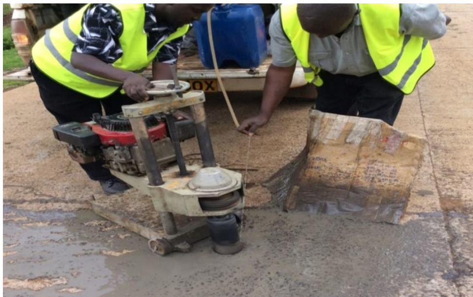
Figure 3.4: Core cutting process on concrete slab
