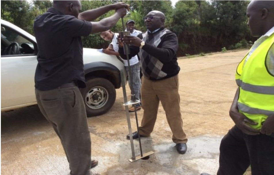
Figure 3.10: Field testing using DCP equipment
