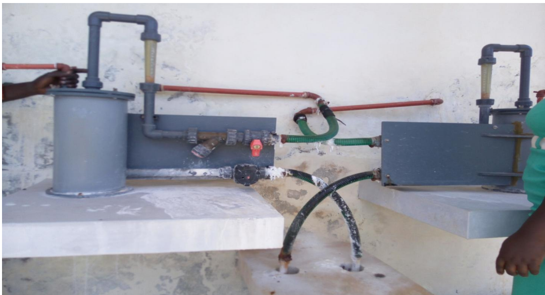
Photo taken at Yala Water Treatment site
