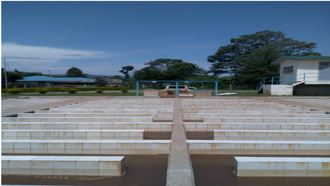
Photo taken at Yala water treatment works
