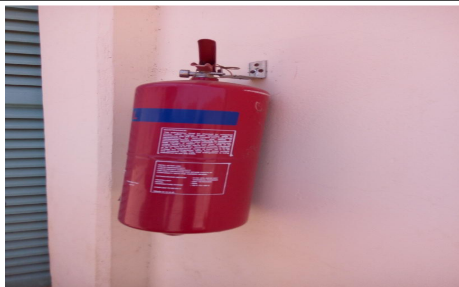
Photo taken at KIWASCO Administrative block
