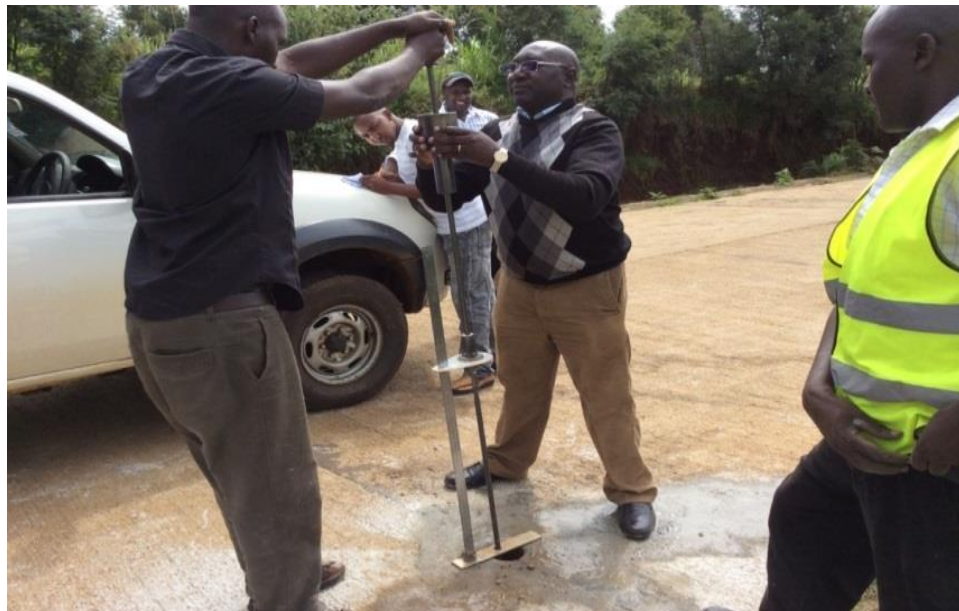
Figure 3.10: Field testing using DCP equipment
