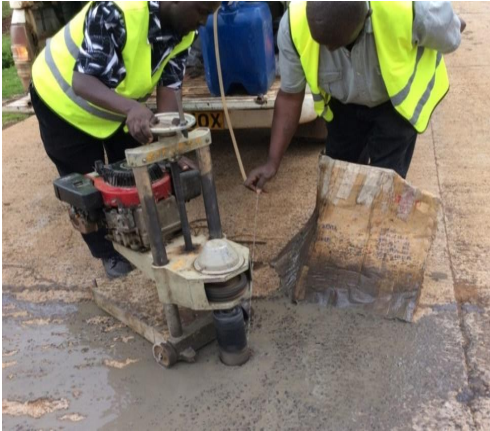
Figure 3.4: Core cutting process on concrete slab
