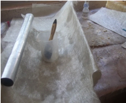
Application of resin and GRF layers
