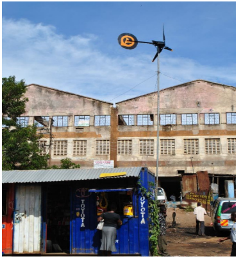
Wind turbine for lighting
