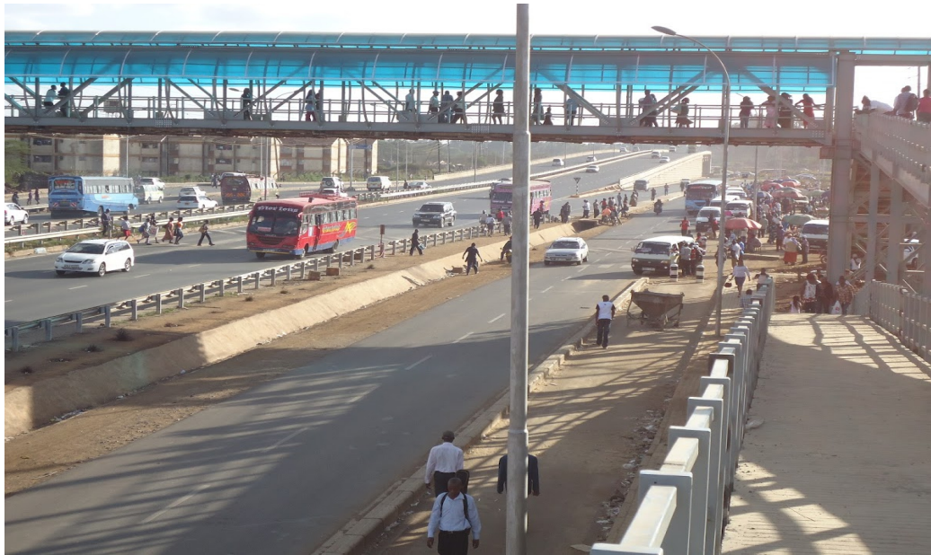
Figure 4.13: Pedestrians Using Foot Bridge at Kasarani
