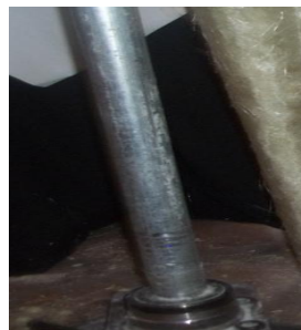
Pipe & car bearing fitted among others
