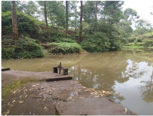
(a) Intake weir
