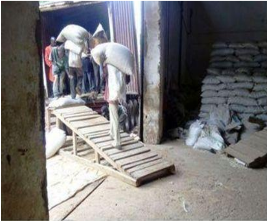
Plate 4.3: Workers involved in carrying of heavy load
