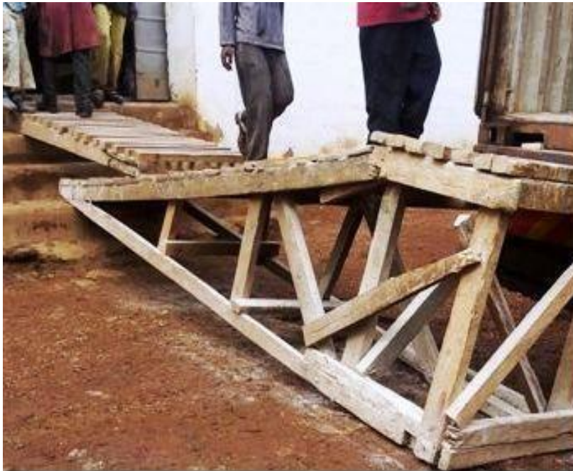
Plate 4.5: Unsafe working platform
