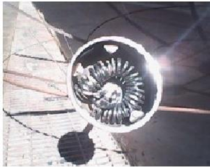
Plate 2.3: Construction of Absorber before enclosing it
