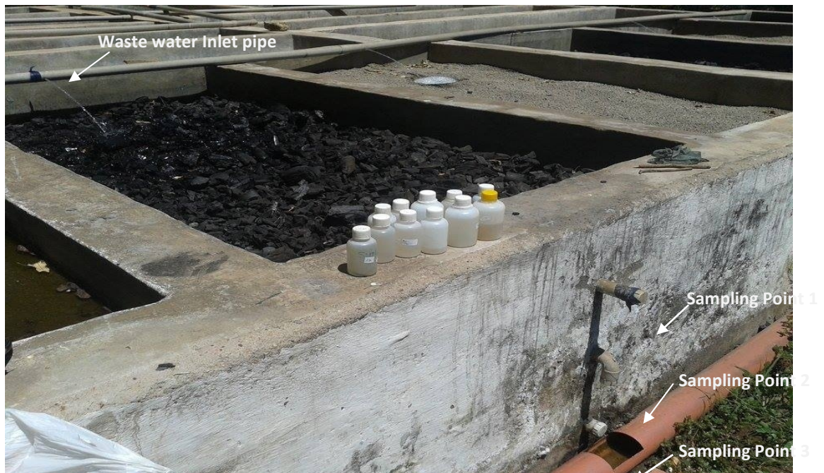
Figure 3-9: Photo showing the inlet pipe of the treatment cells, the sampling points and drainage pipes.
