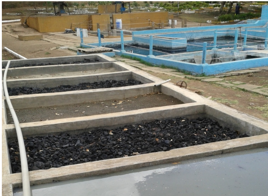
Figure 3-7: Constructed adsorbent beds filled with pumice and charcoal
