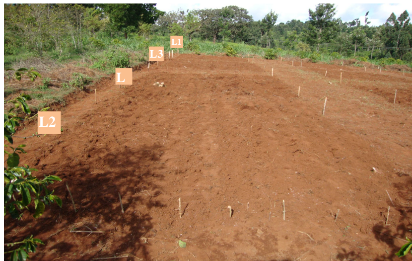
Plate 2: Site appearance after mixing the lime with the soil
