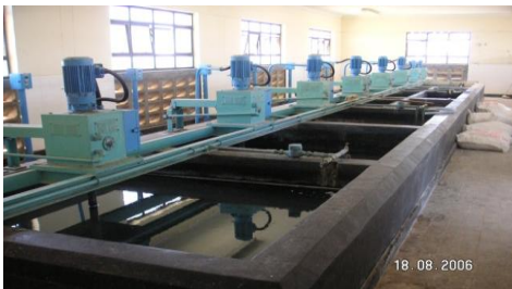
Upper Malewa Treatment works
