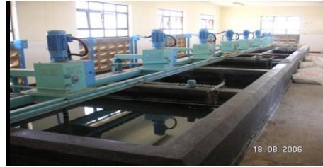
Turasha Treatment works
