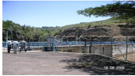
Turasha intake point (Upstream of Turasha
