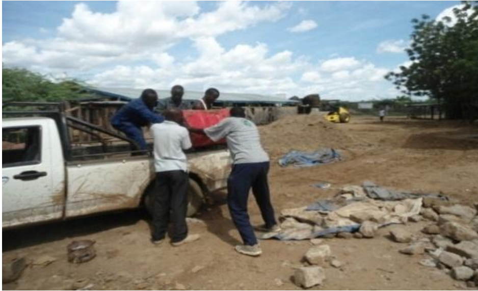
Fig. 8-2 Off-Loading Used Lube Oil for Use at the Site
