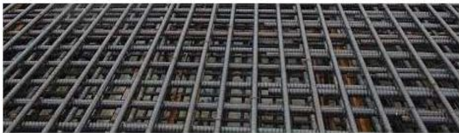
Figure 2.3: Typical Welded Wire Fabric [13]
