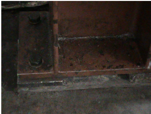
(a) Foot, on rubber pads, secured to floor by rag bolts
