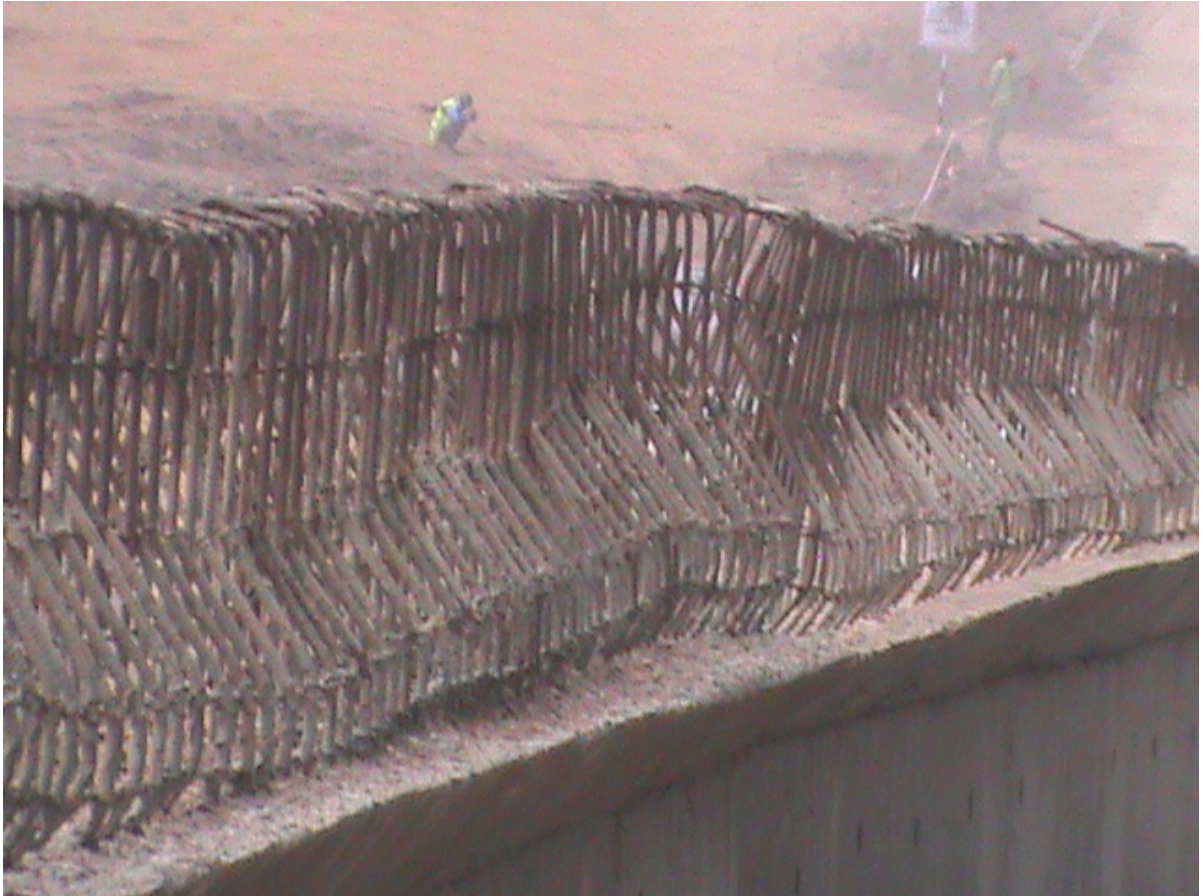
Figure B.1: Bent Bars at a section of Thika-Nairobi highway
