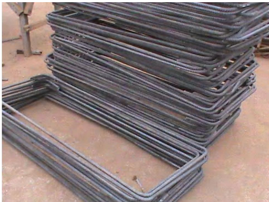
Figure B.7: Bent stirrups for the Nairobi-Thika highway using the above bender, (SHENG-LI Co., Mang'u site)
