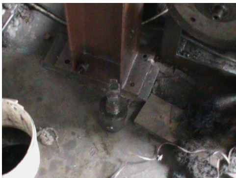
(a) Machine footing floating on timber
