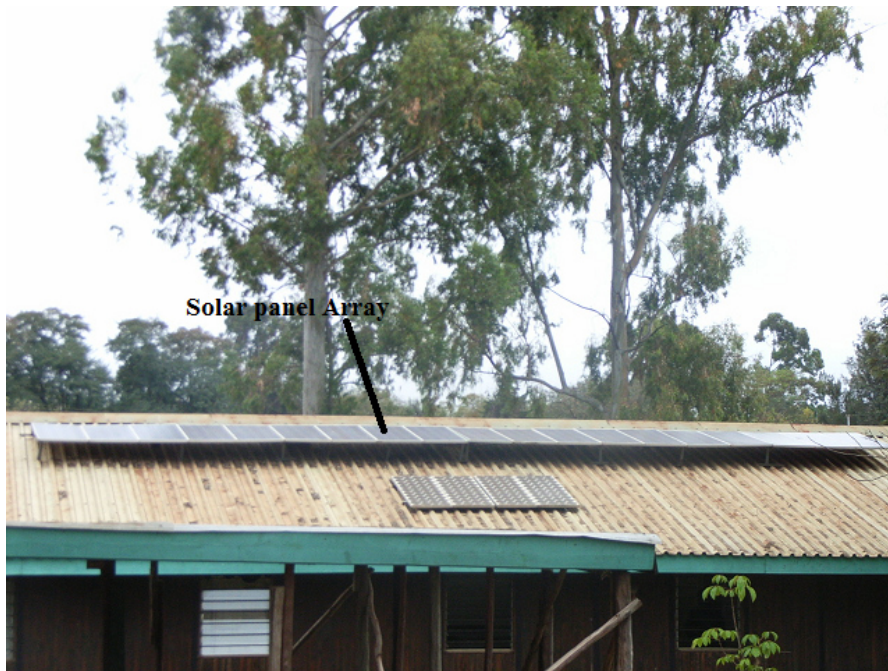
Plate 4 19 solar panel array at the renewable energy centre
