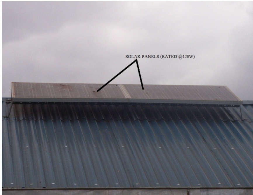
Plate 5 The 2 solar panels installed in a house in Ruiru.
