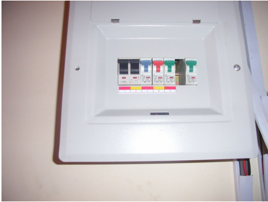
Plate 7 The distribution unit for a PV system for the house in Ruiru
