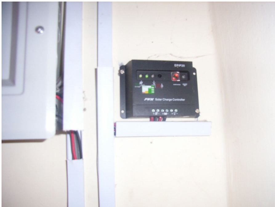
Plate 8 Charge controller for a house in Ruiru
