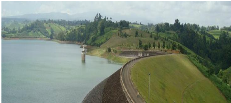
Fig 2.3Thika Dam (Source: NAWASCO, 2011)
