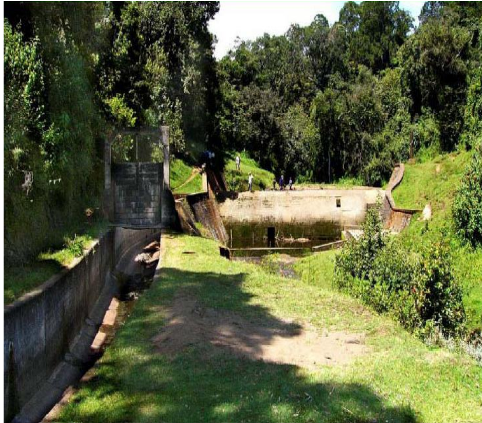
Fig 2.2 Sasumua Treatment Plant (Source: NAWASCO, 2007.)
