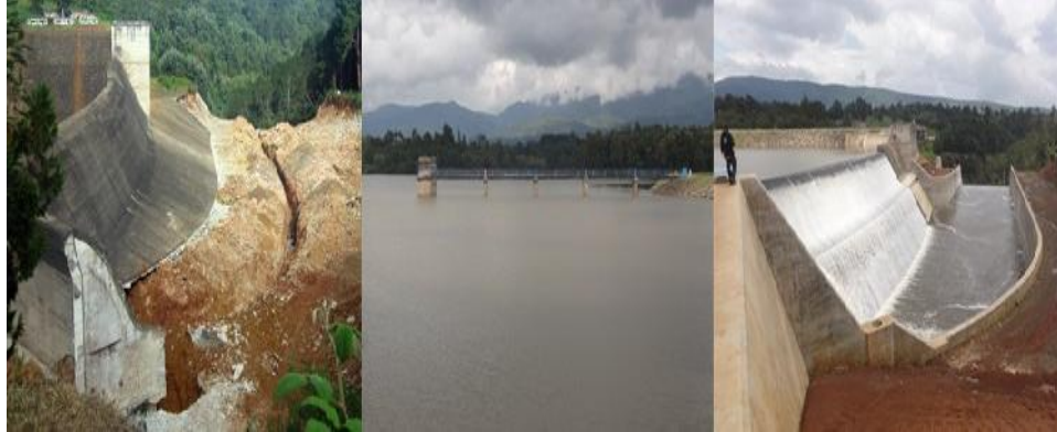
Fig 2.1 Sasumua Dam (Source: NAWASCO, 2011)
