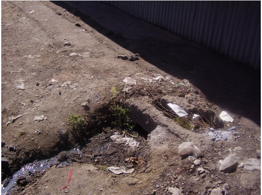
Figure 2. A picture showing a burst sewer in Slota area, Athi-River.
