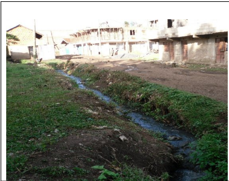
Figure 3: Domestic wastewater flowing in open ditches which finally discharge into Kiu River
