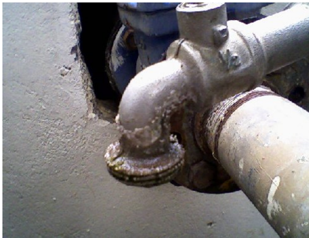
Figure 2: Corrosion of pipes in HACO Industries, Kasarani
